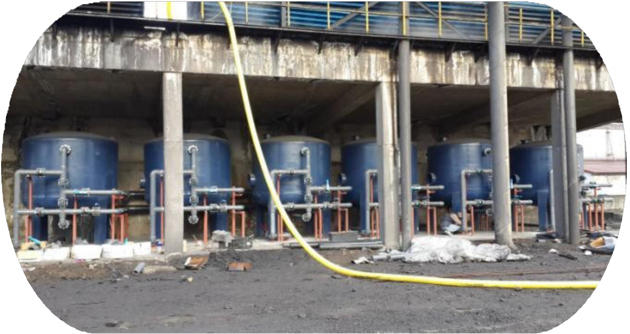
MAKE-UP WATER PREPARATION UNIT RO + PRETREATMENT Capacity : 200 m 3 /h
