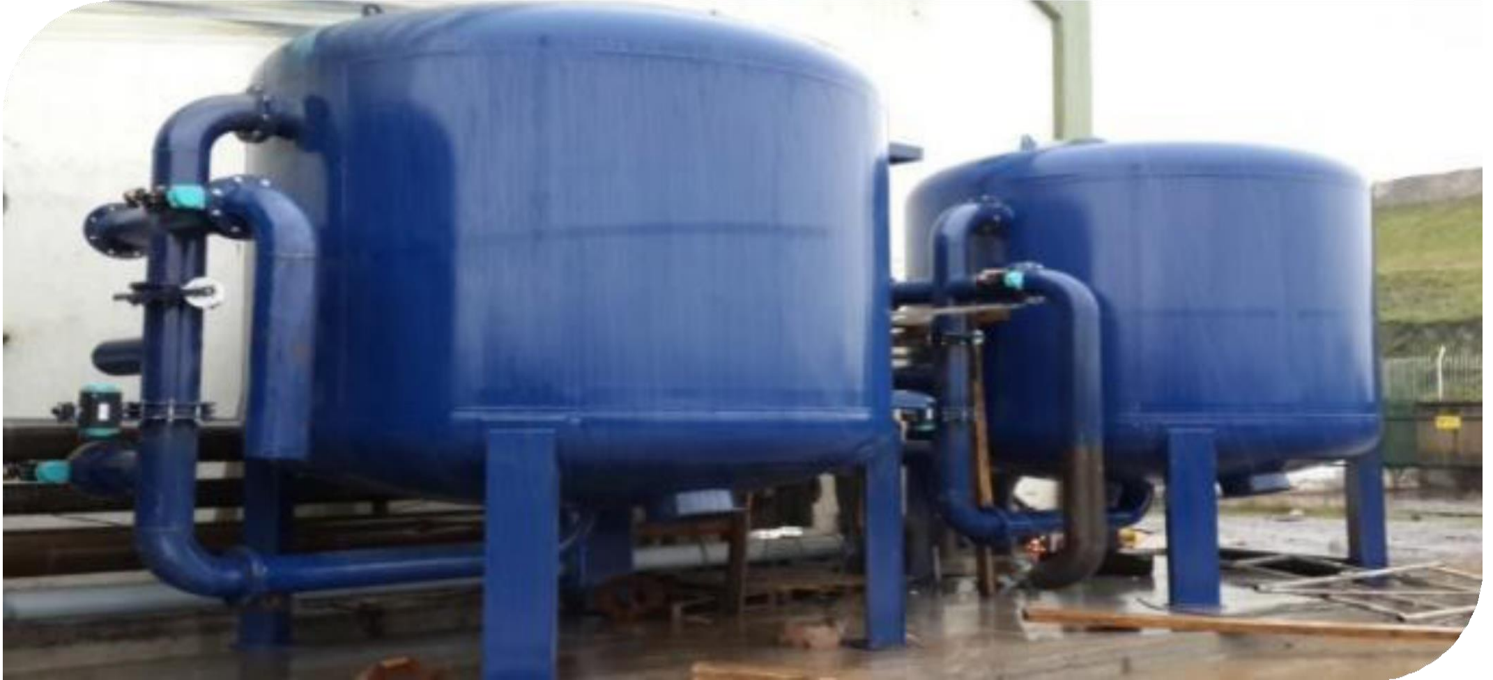
CCM DIRECT COOLING CIRCUIT 500 m 3 /h
