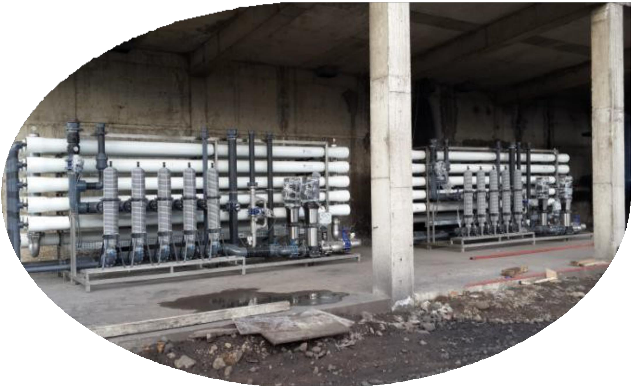
MAKE-UP WATER PREPARATION UNIT RO + PRETREATMENT Capacity : 200 m 3 /h
