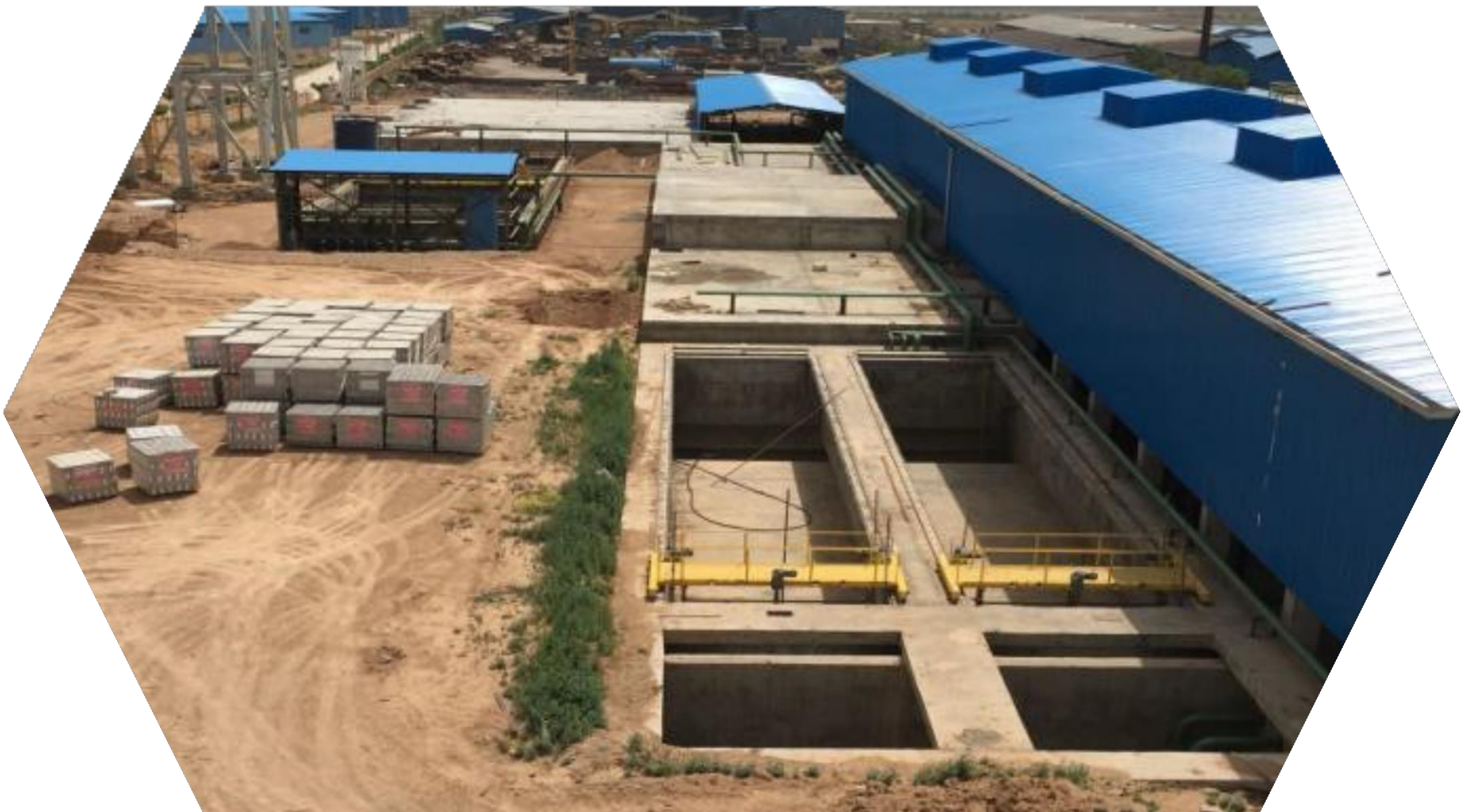
SEDIMENTATION TANK THICKNER DAF UNIT
