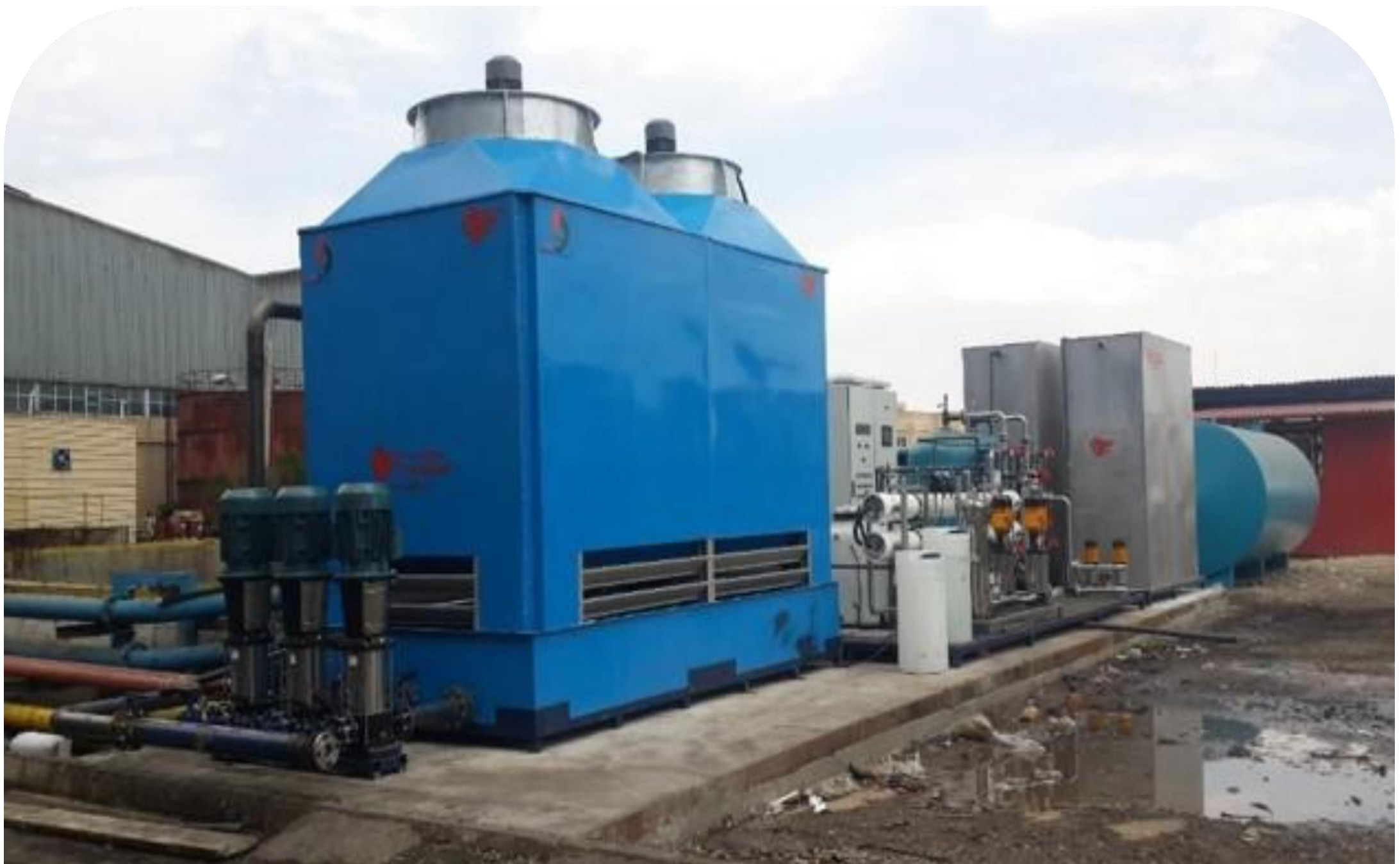
CLOSED CIRCUIT COOLING SYSTEM CAPACITY : 960 m 3 /day
