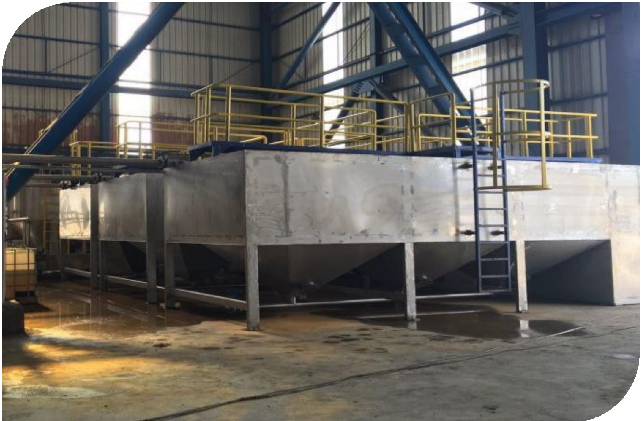
CAPACITY: 1500 m 3 /day LAMELLA SYSTEM
