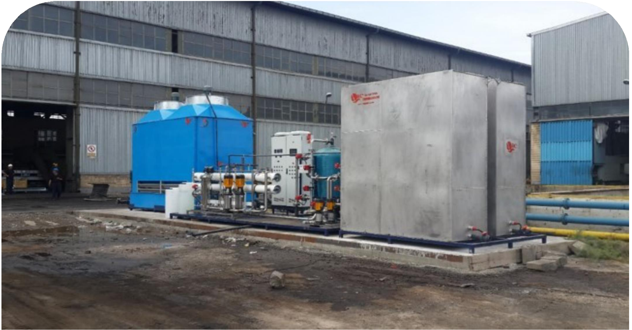
CLOSED CIRCUIT COOLING SYSTEM CAPACITY : 960 m 3 /day
