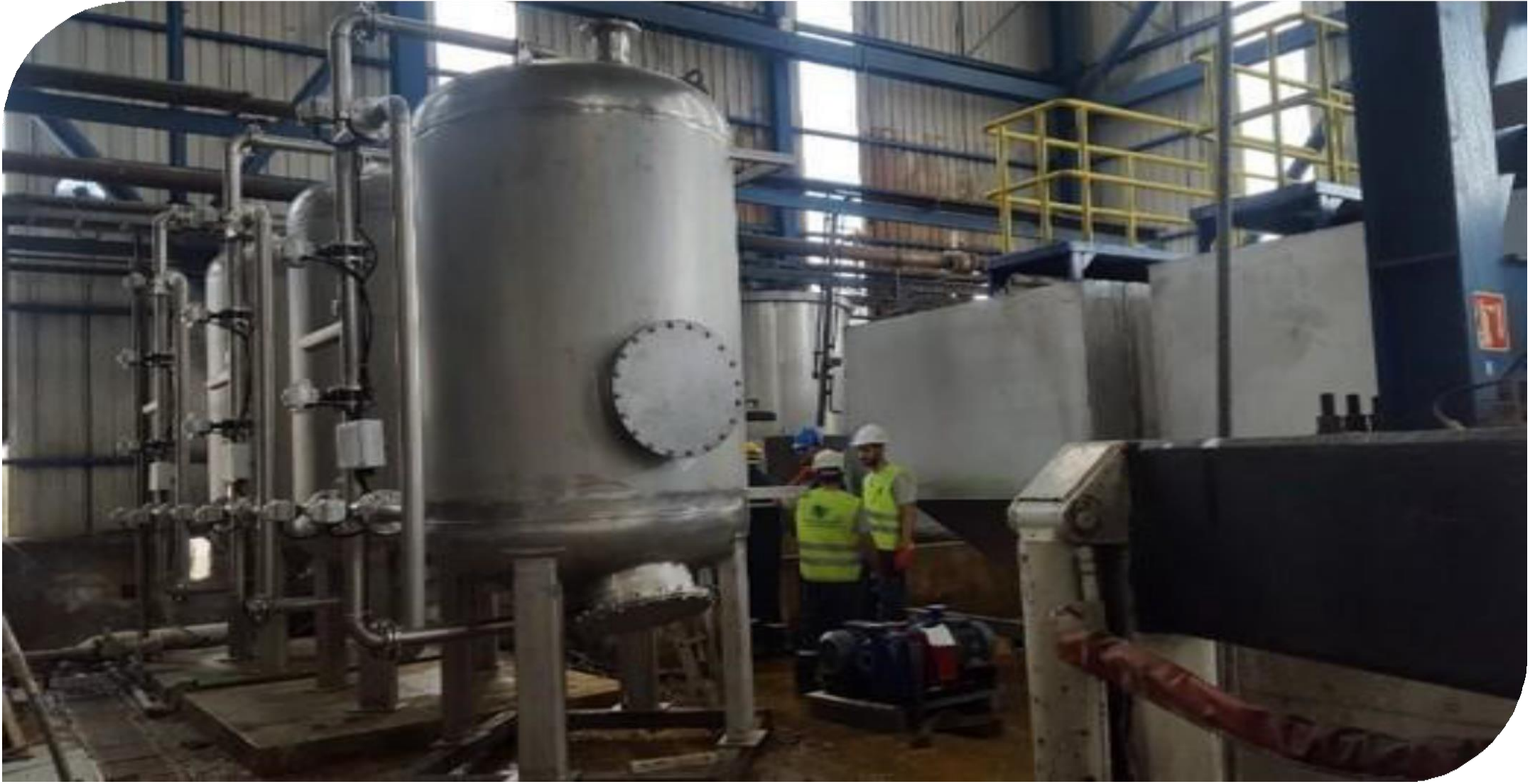
CAPACITY: 1500 m 3 /day LAMELLA SYSTEM
